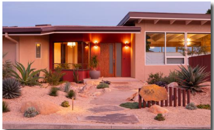
ARROYO SECO CONSTRUCTION won the Design/Build Award for the La Vista Grande project.
