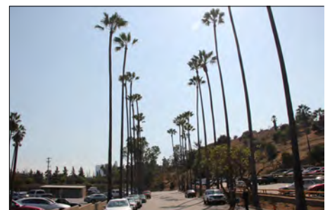
FINISHED PROJECT sports a fresh, clean look for the street and adjacent areas leading up to the Police Academy entrance. Many thanks to all those companies and individuals who made it possible.
